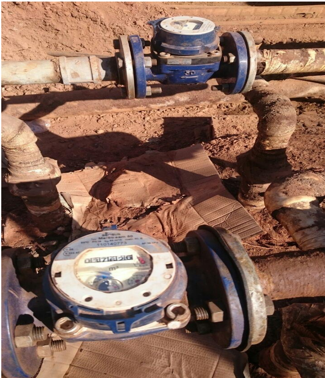
Old water meters being removed. Note the condition of the pipe below
